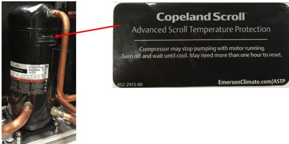
Figure 20: Advanced Scroll Temperature Protection (ASTP)
