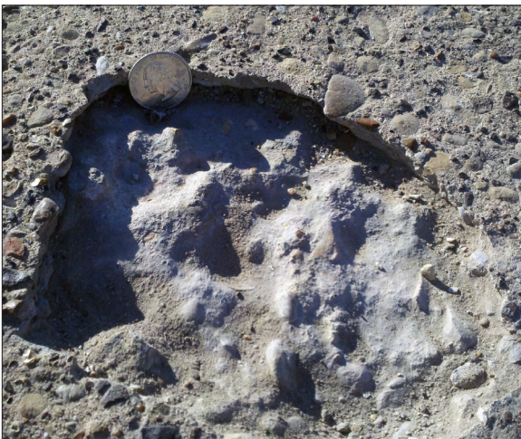
Pit in concrete
