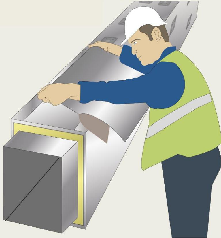
*Figure 13 shows the installer lining up the 3M™ VentureClad™ top sheet with the duct's edges (piece 4). After being installed, this sheet of 3M™ VentureClad™ should overlap each vertical side by 3 inches (75mm).*
