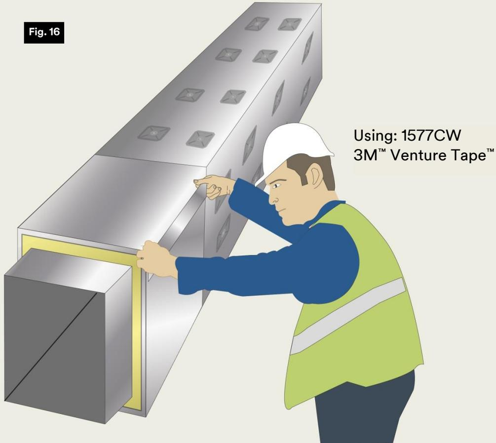
*Figure 16 shows the cut strip of 4 inch (100mm) wide 1577CW 3M™ Venture Tape™ being applied to reinforce a joint when using 1579GCW 3M™ VentureClad™. Be certain to run over the tape with a squeegee after applying it to the 3M™ VentureClad seam. Note that the more flexible 1578CW 3M™ Venture Tape™ may also be used to seal the 3M™ VentureClad™ seams.*
