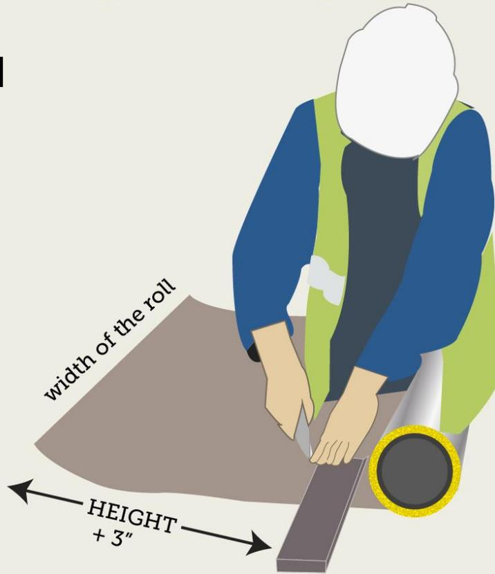
Figure 8 shows the installer cutting his second sheet (piece 2 or 3) of 3M™ VentureClad™, this one to be applied to one of the two vertical sides. Note that its minimum dimension is equal to the insulated duct height + 3 inches (75mm).
