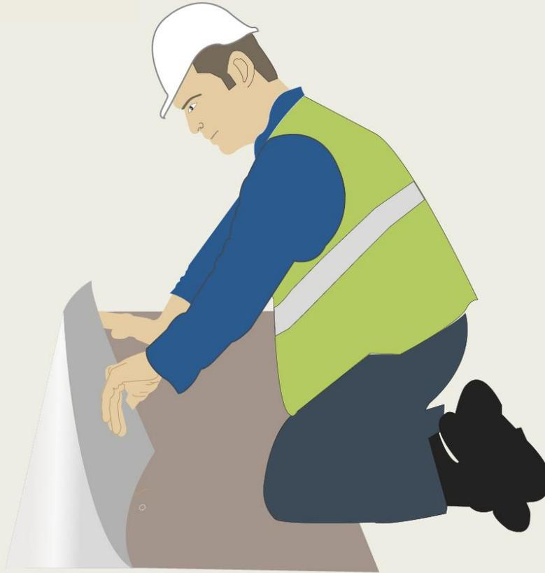
*Figure 5 shows the installer starting to remove the release liner to expose the pressure sensitive adhesive. He should only pull the release liner back 3–4 inches (75–100mm), then start applying it to the face of the insulated duct, as shown in Figure 6.*
