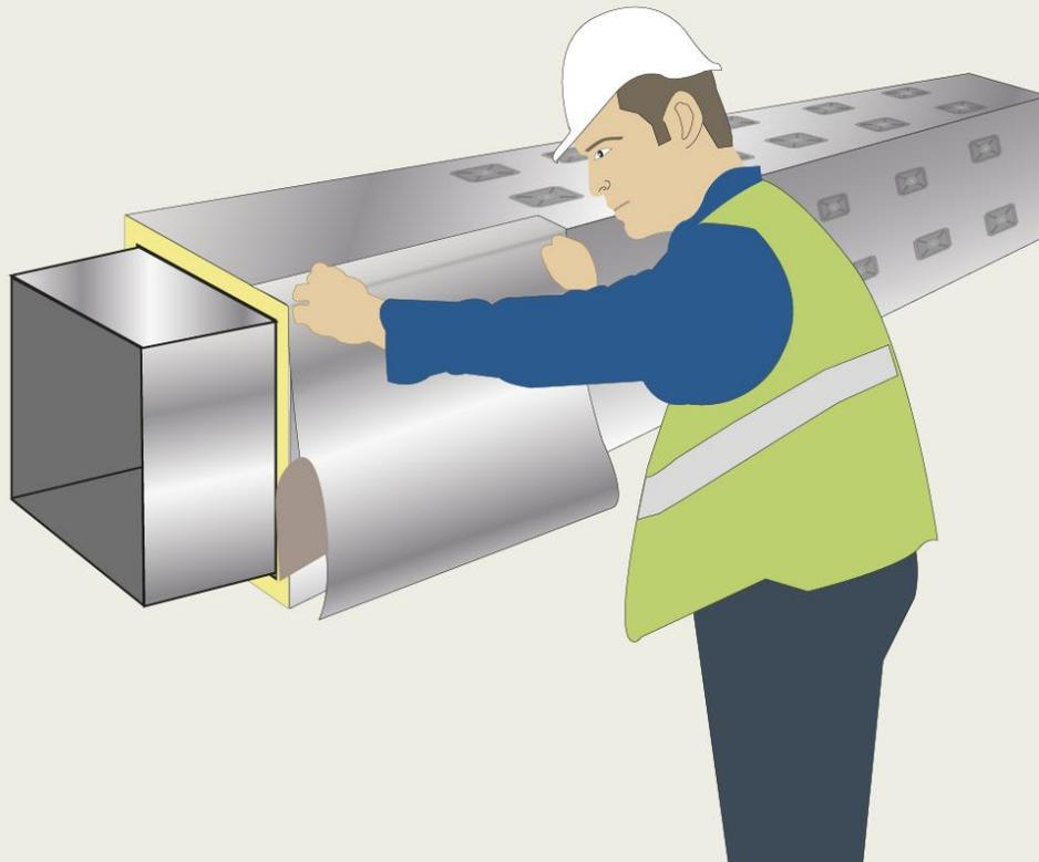
*Figure 9 shows the installer applying the cut sheet of 3M™ VentureClad™ to the vertical side (piece 2). Note that he first lines up the top edge of the 3M™ VentureClad™ with the top edge of the insulated duct, then works his way down the side, peeling back the release liner in steps, then applying that section with the exposed adhesive.*
