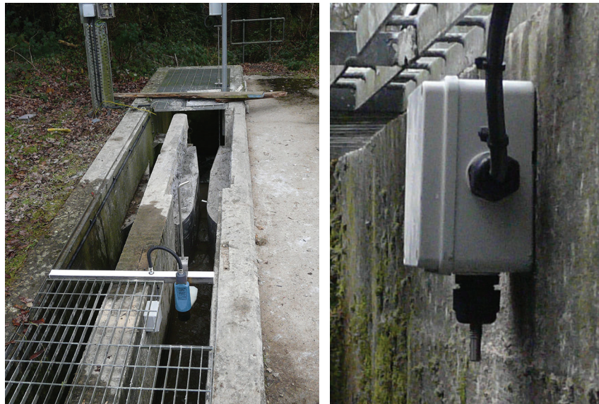
Figure 3-7. Enclosed or partially covered flume chamber arrangement
