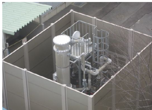
Groundwater purification equipment at the headquarters office
