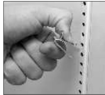
Fig. 1. Installing top tab of shelf clip.
