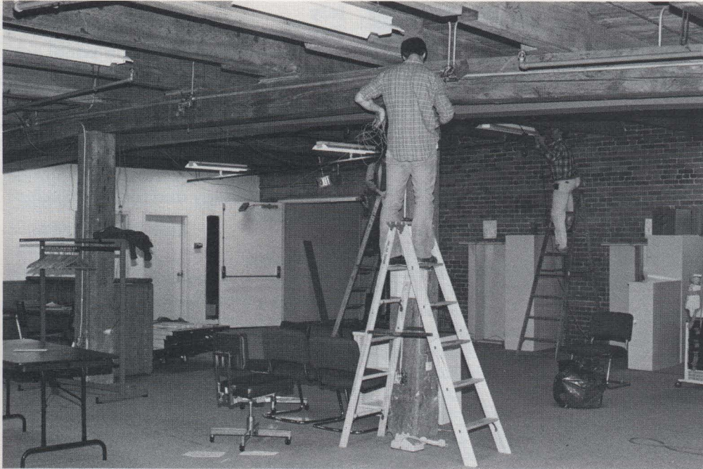
Office Preparations. Before the staff arrives from Marlboro, workers ready the newly renovated office space at Museum Wharf.
