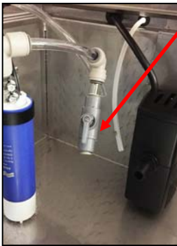
Fig. 3 Priming valve in OPEN position
