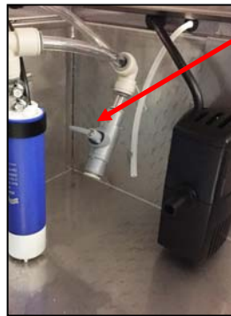
Fig. 3 Priming valve in OPEN position
