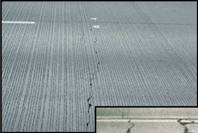
CRC Transverse Cracking
