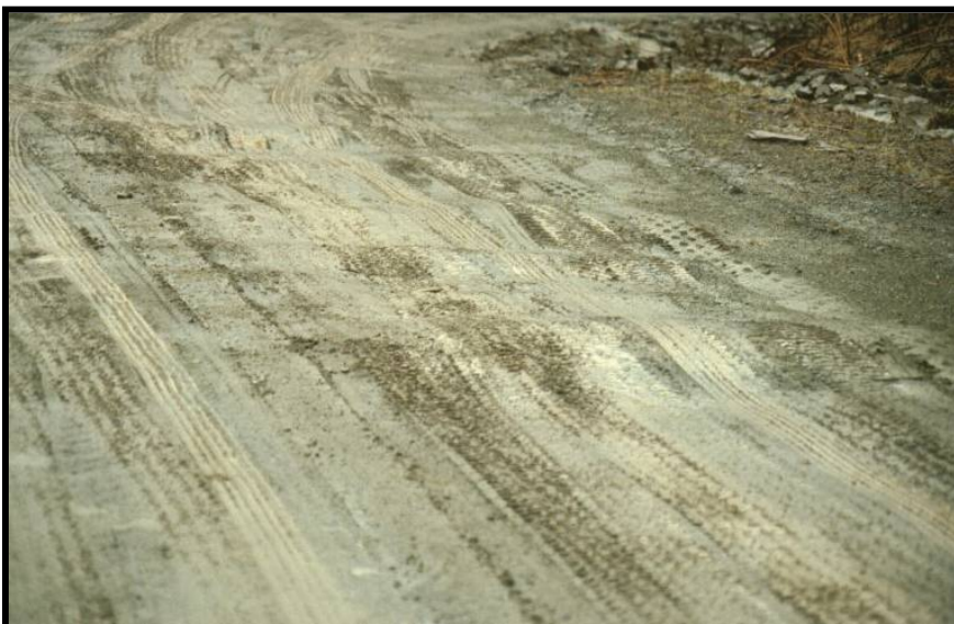
Corrugations – High Severity
