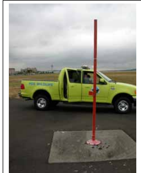
Poles and other structures that are no longer in use should be removed from airport property. Such structures make ideal perching sites for hawks and owls searching for prey. The pellets at the base of this pole are undigested fur and bones of rodents that were regurgitated by red-tailed hawks (photo by R. A. Dolbeer, USDA).
