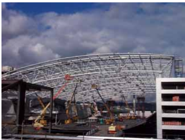
Within 2 weeks of completion, starlings and pigeons had started roosting in this canopy constructed over the passenger drop-off area at a major USA airport (photo by S. Gordon).
