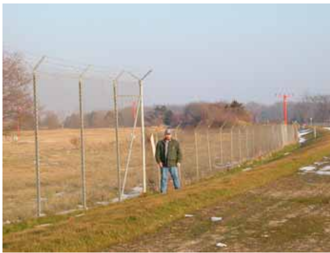
A well-maintained fence, at least 10-feet high with no gaps at the bottom, is the primary defense to keep deer and other large animals off the airport's AOA. Deer can easily jump fences that are only 6 feet high (right) (photo by R. A. Dolbeer, USDA).
