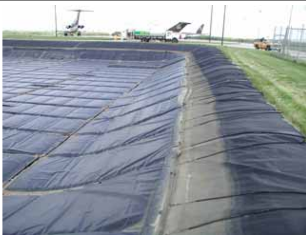
Birds are permanently excluded from this storm water detention facility through the use of a floating permeable barrier (Photo courtesy Industrial & Environmental Concepts, Inc.).
