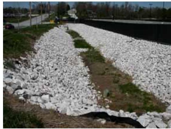
Water detention basins at airports, such as this French-drain system at an eastern USA airport, should be designed to completely drain within 48 hours after the design storm event (photo by R. A. Dolbeer, USDA).
