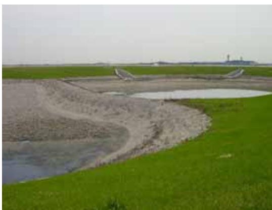
This storm water basin was designed to drain within 48 hours following a major storm event (the design storm). The rip-rap lining helps prevent vegetation growth and bird use of the pond (photo courtesy FAA).
