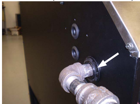
FIGURE 28 - FURNACE GAS PIPE CONNECTIONS (NOTE RUBBER GROMMET)
