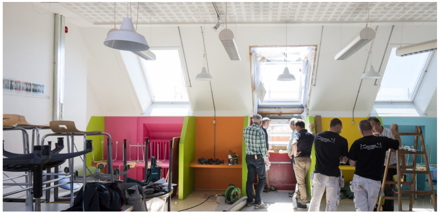
Installation phase of the roof windows
