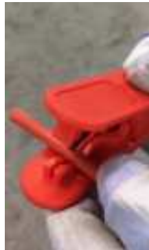
Figure 10-18 Cutting off the end of the fire-trace tube
