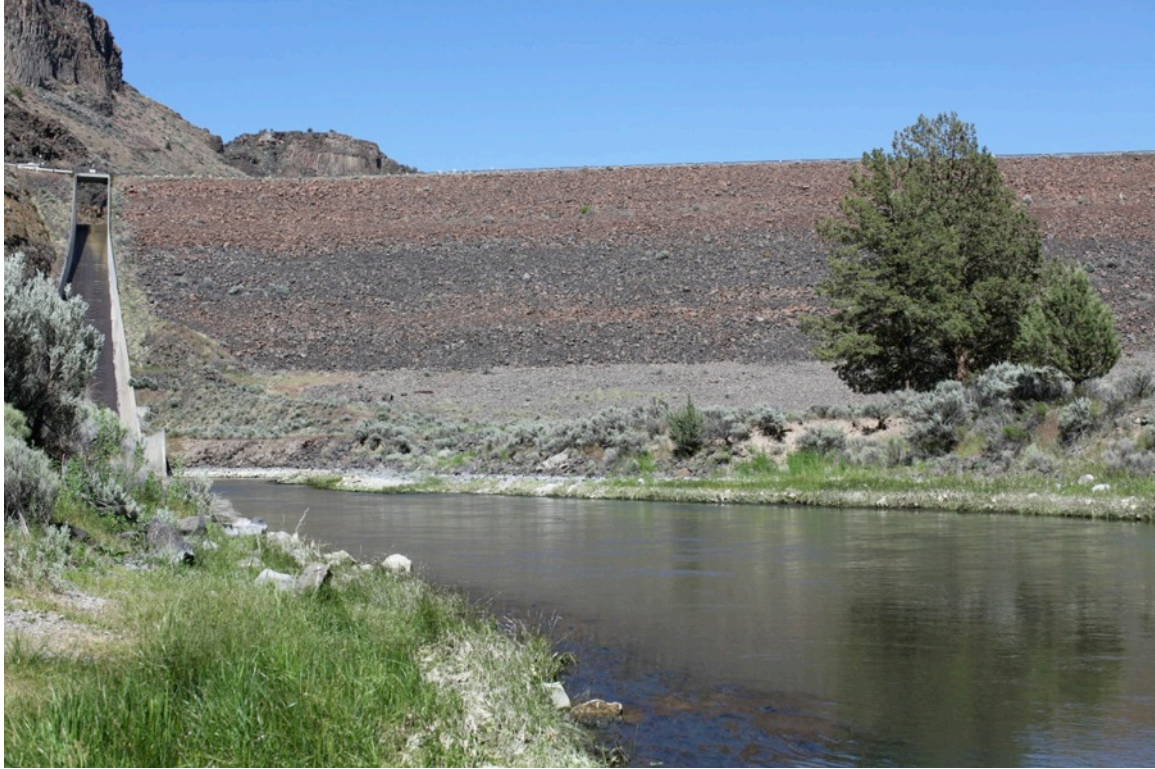
Bowman Dam East dam retaining wall
