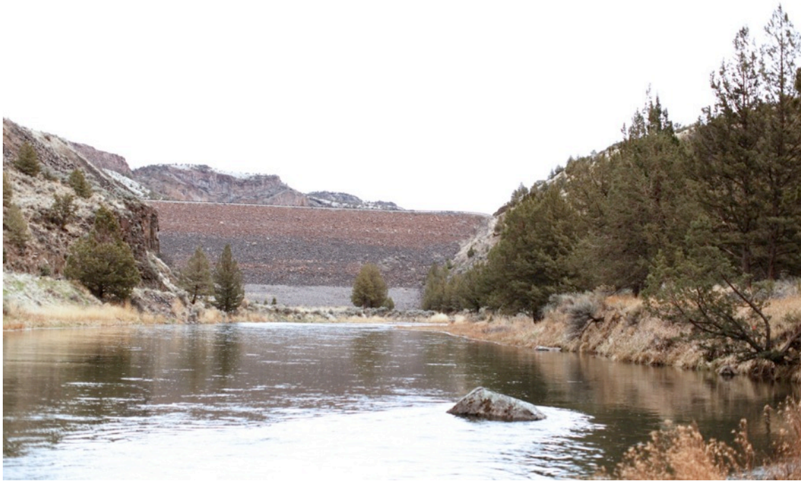
Bowman Dam East dam retaining wall view from downstream
