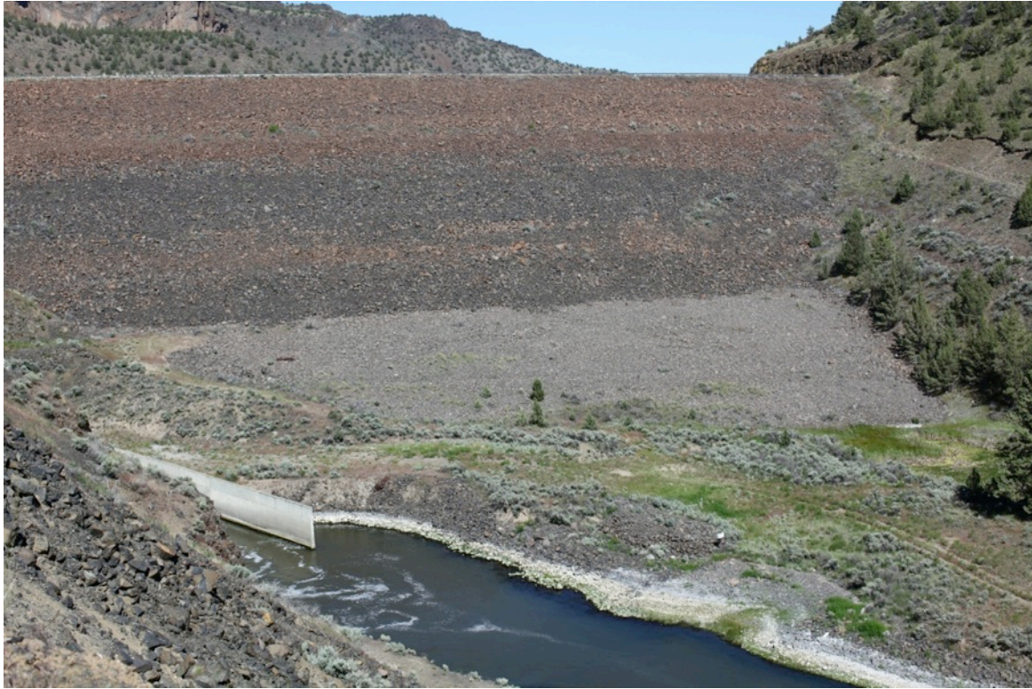
Bowman Dam East dam retaining wall upper view
