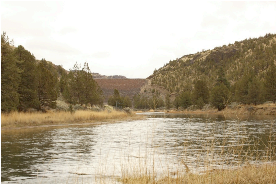
Bowman Dam Downstream east view
