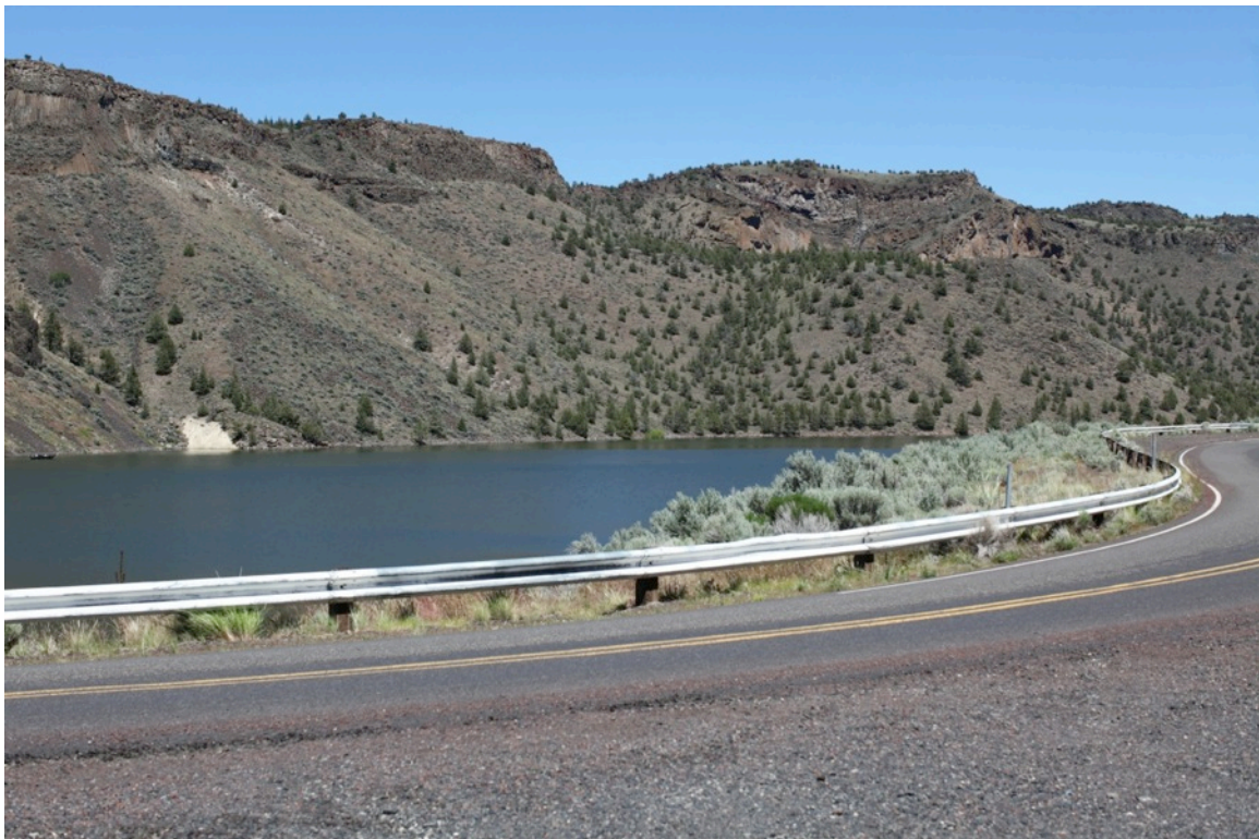
Bowman Dam Reservoir East view above dam
