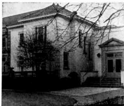
Engineering Club Building, Cincinnati, Ohio
