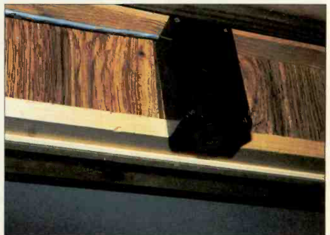
Photo 1b: The circuit in photo 1a enclosed in a box over a doorway to detect people or small animals walking through it.
