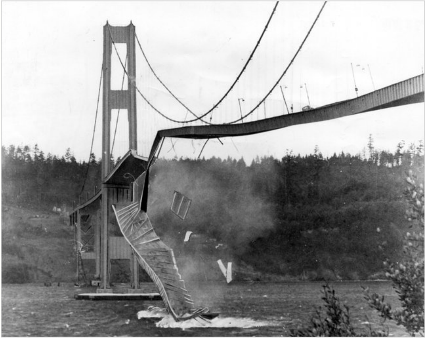
Avoiding perverse outcomes: The Tacoma-Narrows bridge, located in the northwestern part of the United States, collapsed because small vibrations in the wind resonated with the bridge's natural frequency. This created an amplifying oscillation that ultimately led to a catastrophic collapse. (Photo: Associated Press; NYT July 19, 2010).
