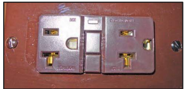
Figure 9-9: GFCI Receptacle
