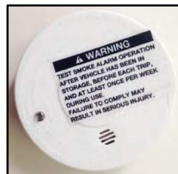
Figure 2-4: Smoke Detector
