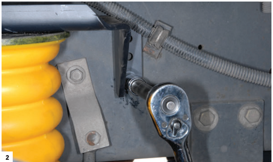
[1] Brackets are bolted to the polyurethane springs before mounting on the motorhome's frame and leaf springs. [2] Existing holes in the frame were used initially to bolt the rear springs into place tightly so the additional holes in the frame could be drilled.
