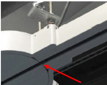
Figure 16 – File the edges of the track
