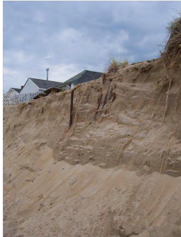
Photograph 1.11. Vertical face of eroded dune showing layering of sediments.
