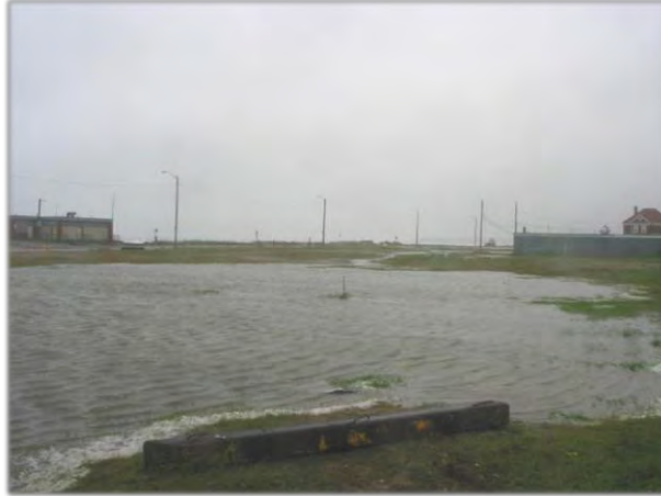
Photograph 2.19. Land subject to coastal storm flowage (and altered dune) with ability to detain and slow flood waters. Here, the area that is delineated as land subject to coastal storm flowage (consisting of gravel, portions of asphalt, and vegetation) has the ability to retain, collect, absorb, and slow water as evidenced by the extensive pool of storm-wave overwash and flood waters that collected after a storm event. If this area were to be developed with solid foundation walls, filled, or paved, the ability of the land to detain and slow the flood waters would be severely diminished, ultimately affecting adjacent properties. The photograph is taken looking toward the ocean (in distance).
