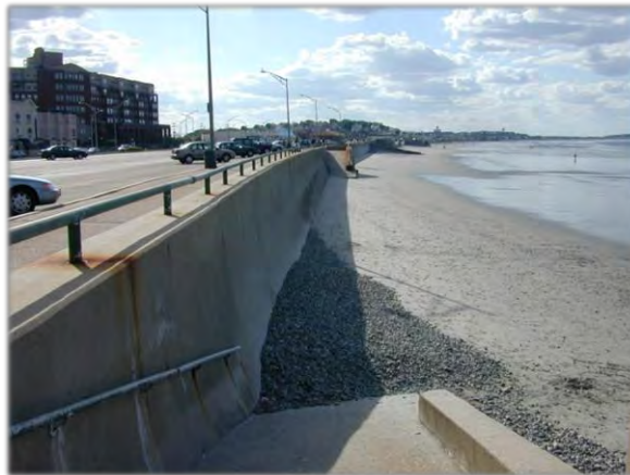
Photograph 2.3. Coastal beach with seawall. In spite of the seawall, this coastal beach is able to both shift and change form in response to waves and tides and to transport sediment along the shore. There is no longer a dune to serve as a reservoir of sediment for the beach.
