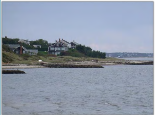
Photograph 2.2. Coastal beach with groins. The groins on this beach disrupt some longshore sediment transport and cause scour of the beach adjacent to each groin. However, they do not completely impede all sedimentary functions, such as the exchange of sand between the dunes, beaches, and subtidal areas of each groin cell.
