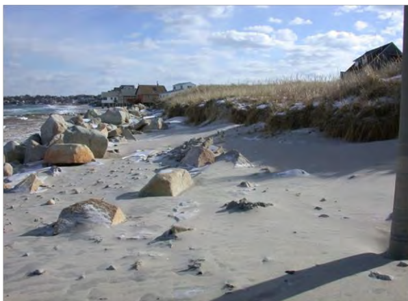
Photograph 1.16: Storm erosion as seen on an eroded scarp on a coastal dune behind riprap. Windblown sand deposition in front of the scarp occurred subsequent to the storm.
