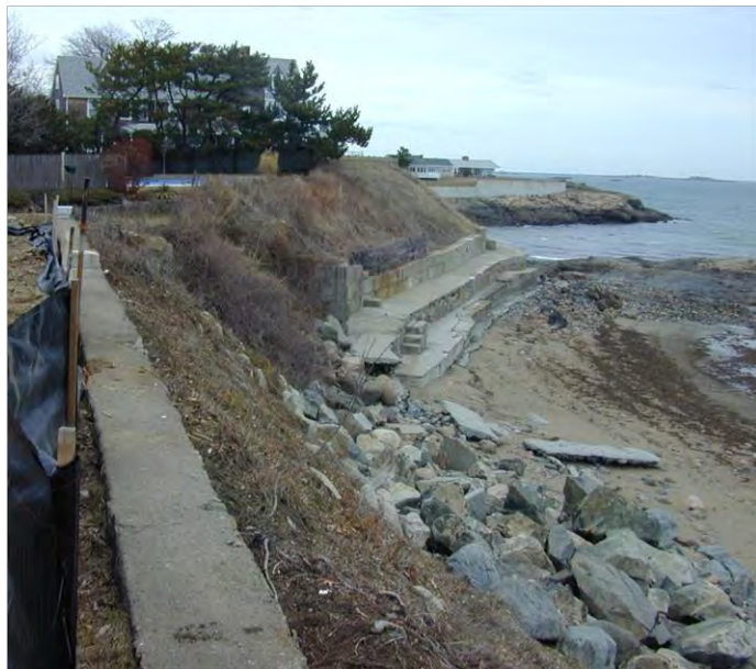
Photograph 4.6. Pre-existing riprap on coastal bank and coastal beach. The rocky intertidal shore can be seen in the distance.
