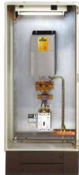
DC590+ DRV equivalent illustrating panel space saving
