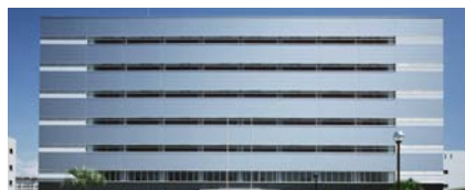
Advanced Technology R&D Center (Amagasaki, Hyogo)
