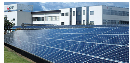
Power Distribution Systems Center (Marugame, Kagawa)
