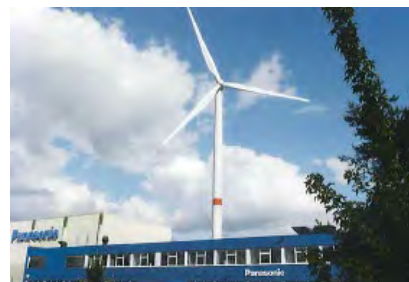
Wind power generation system in PECBE
