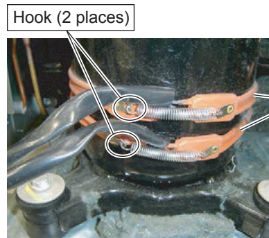
Crank Case Heater (2 places)
