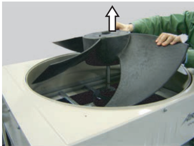
Remove the Propeller fan. Note at the installation. Insert propeller fan and motor shaft reference D cutting position.
