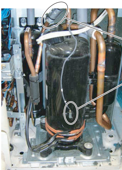
Discharge temp. thermistor (TH1)
