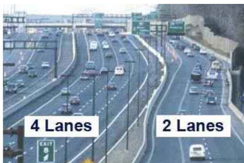
Figure 3 Enter the total through lanes in both directions, excluding designated turn lanes.
