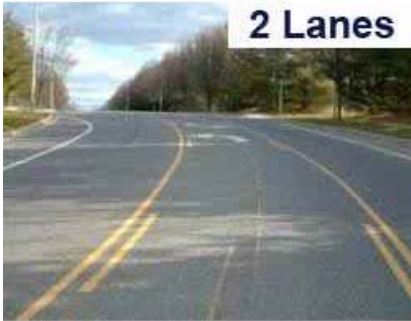
Figure 5 Enter the total through lanes in both directions, excluding designated turn lanes.
