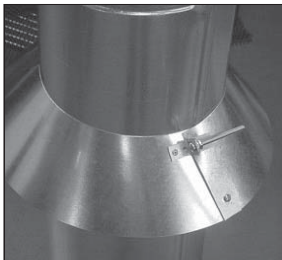
Figure 8.17 Assembling the Storm Collar Around the Pipe
