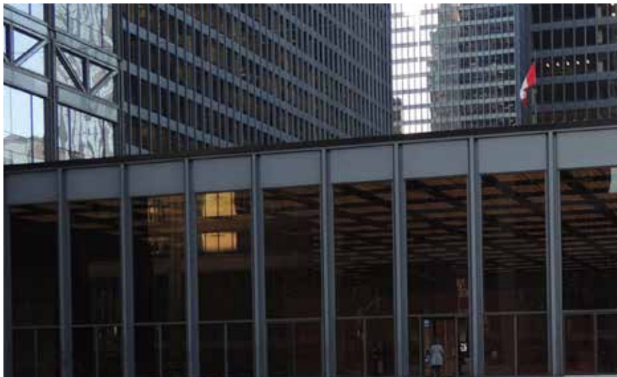
Unacceptable to use Tinted Glass
