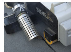
Modified bitumen welding
