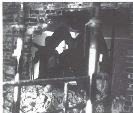
Dixon's workmen open up the brick wall.
