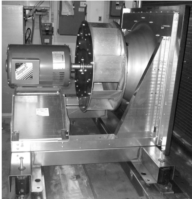
Figure 1. eDrive™ direct-drive plenum fan
