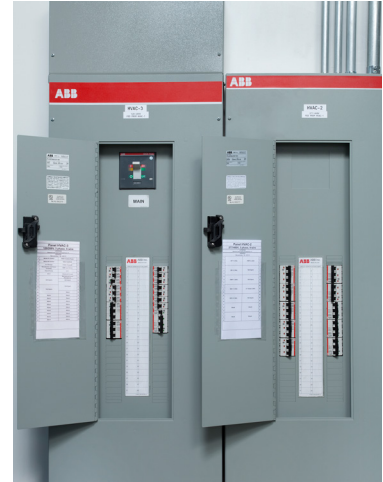
ProLine Panelboard installed in the VPP rated ABB, New Berlin facility
