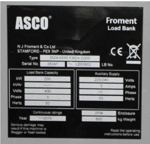
Figure 2-2 Consult the load bank’s name plate for voltage and current ratings before making connections
