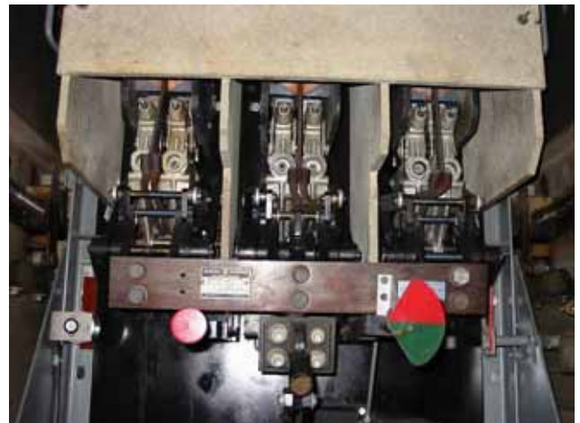
Figure 5. High resolution IR image and visual photo of 480 volt generator tie-in breaker.
