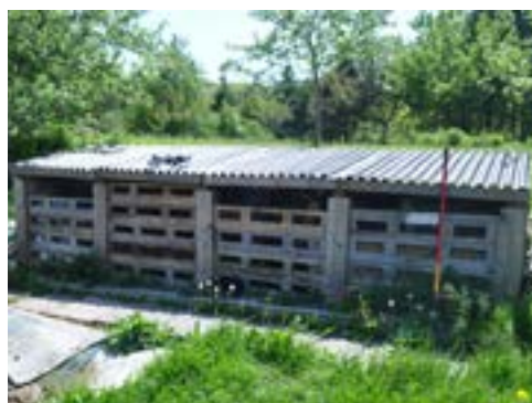
Cement Bins, Spring 2012
