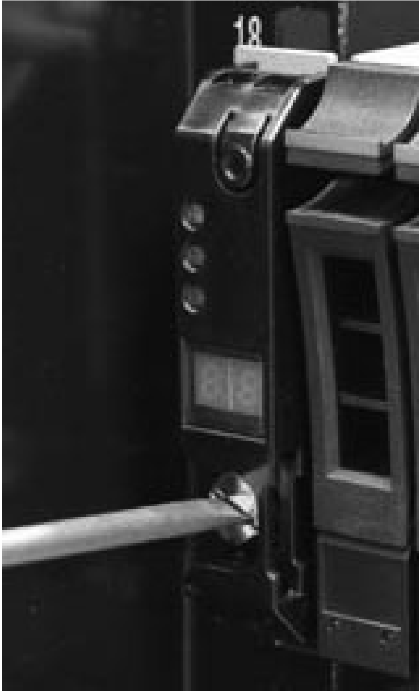
Figure 11. Securing an enclosure to a rack cabinet
