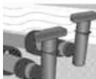
Low Point Drains
