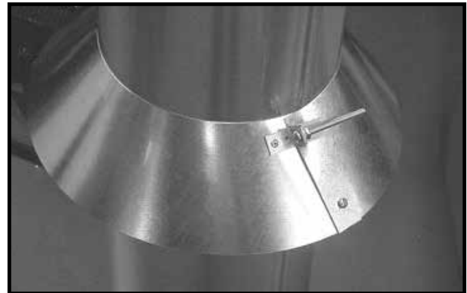
Figure 10.13 Assembling the Storm Collar Around the Pipe
