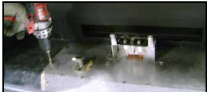
Figure 11.2. Remove Valve Plate Screws
