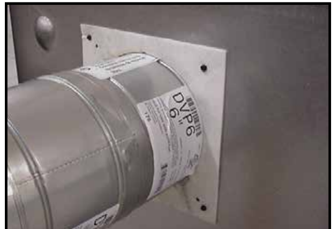
Figure 6.12 Attach the first vent section (it will snap into place). Slide the insulation gasket onto the vent section, up against the appliance and over the tabs. Use four self-tapping screws to secure gasket to outer wrap.
