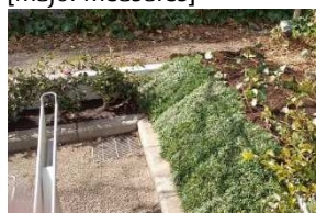
(a) Retaining walls and embankments
