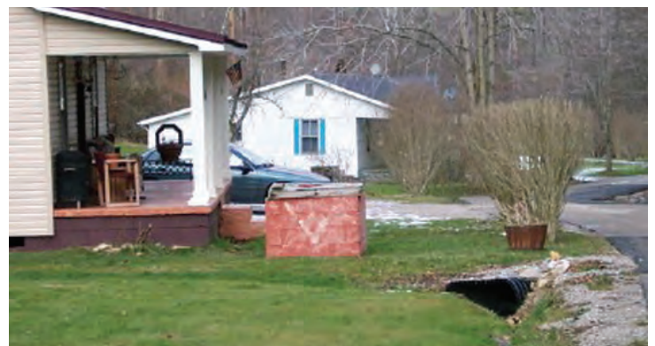
Figure 8.7. Typical Dug Well
