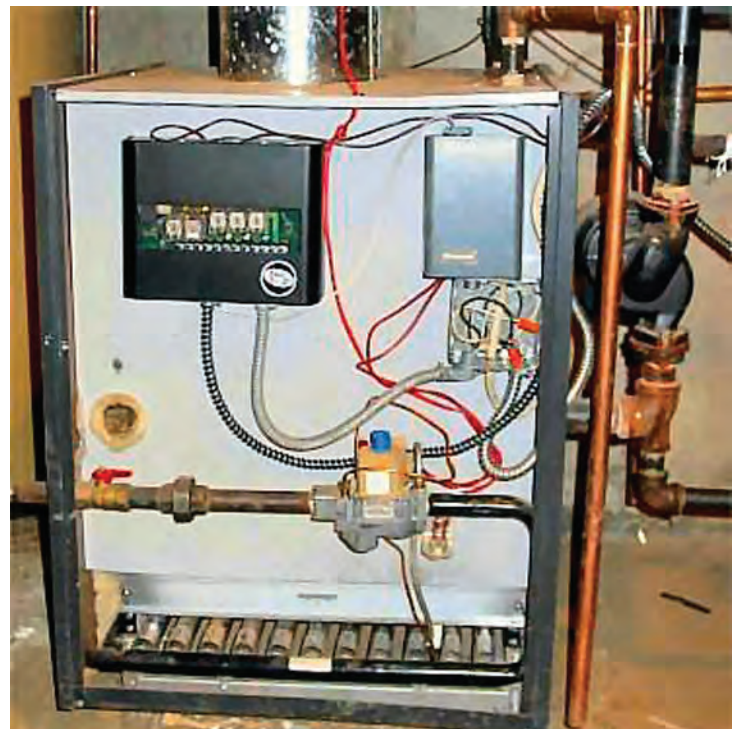
Figure 12.9. Gas-fired Boiler Source: HUD
