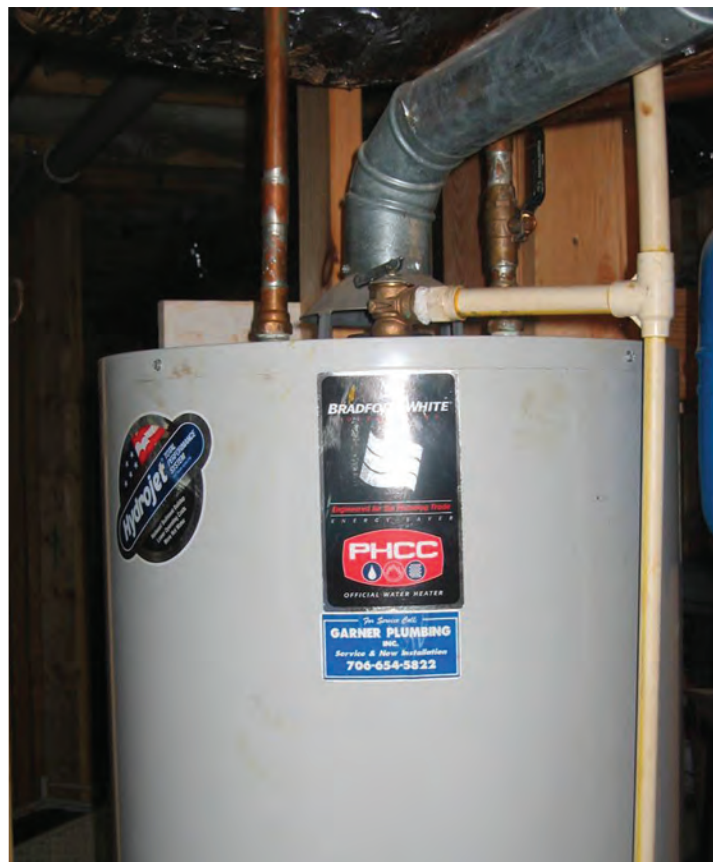
Figure 9.4. Temperature-Pressure Valve
