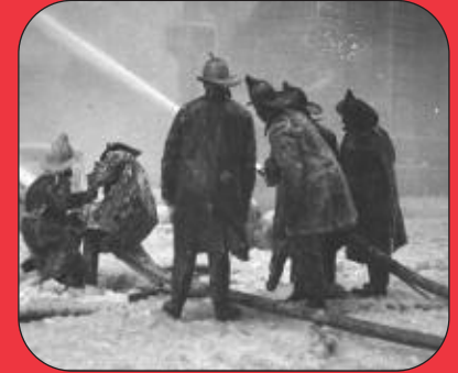
Equitable Building fire, February 1912.
