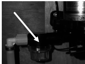
Fig. 8.2 Water pump strainer
