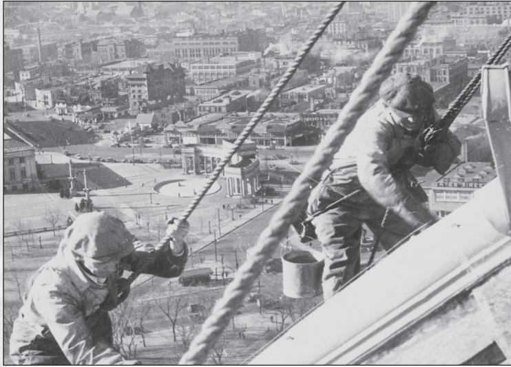
Workmen cleaning and painting the gold dome of the Denver Capitol.
