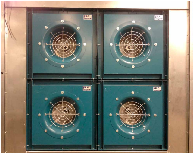
FIGURE 8 - FRONT OF A 2X2 FAN ARRAY
