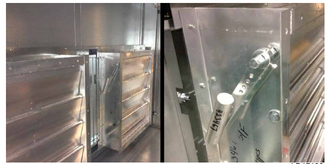
FIGURE 6 - COUNTERBALANCE LOCKED INTO PLACE FOR SHIPPING
