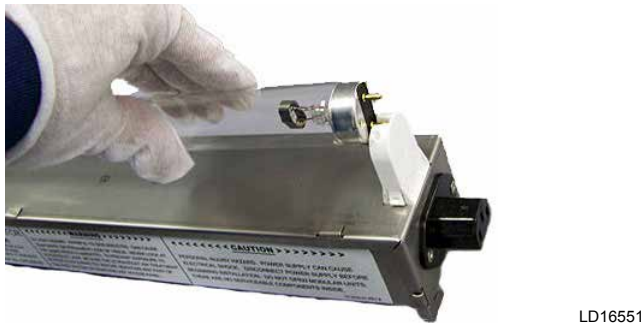
FIGURE 62 - INSTALLING V-MOD LAMP
