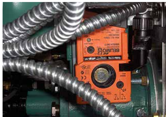
FIGURE 34 - DAMPER ACTUATOR
