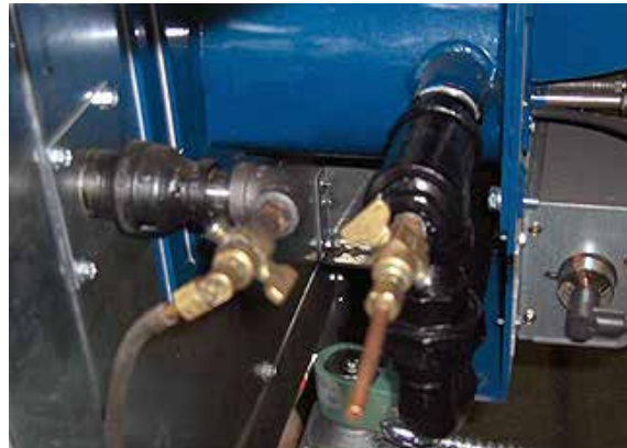
FIGURE 32 - DRAFT OVER FIRE TEST PORT
