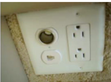
Figure 7-8. 120 VAC Receptacle
