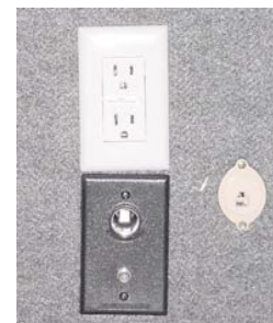
Figure 7-9. 12 VDC Receptacle (black)
