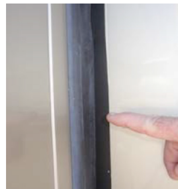
Figure 13-6. Inspecting Slide Out Gasket
