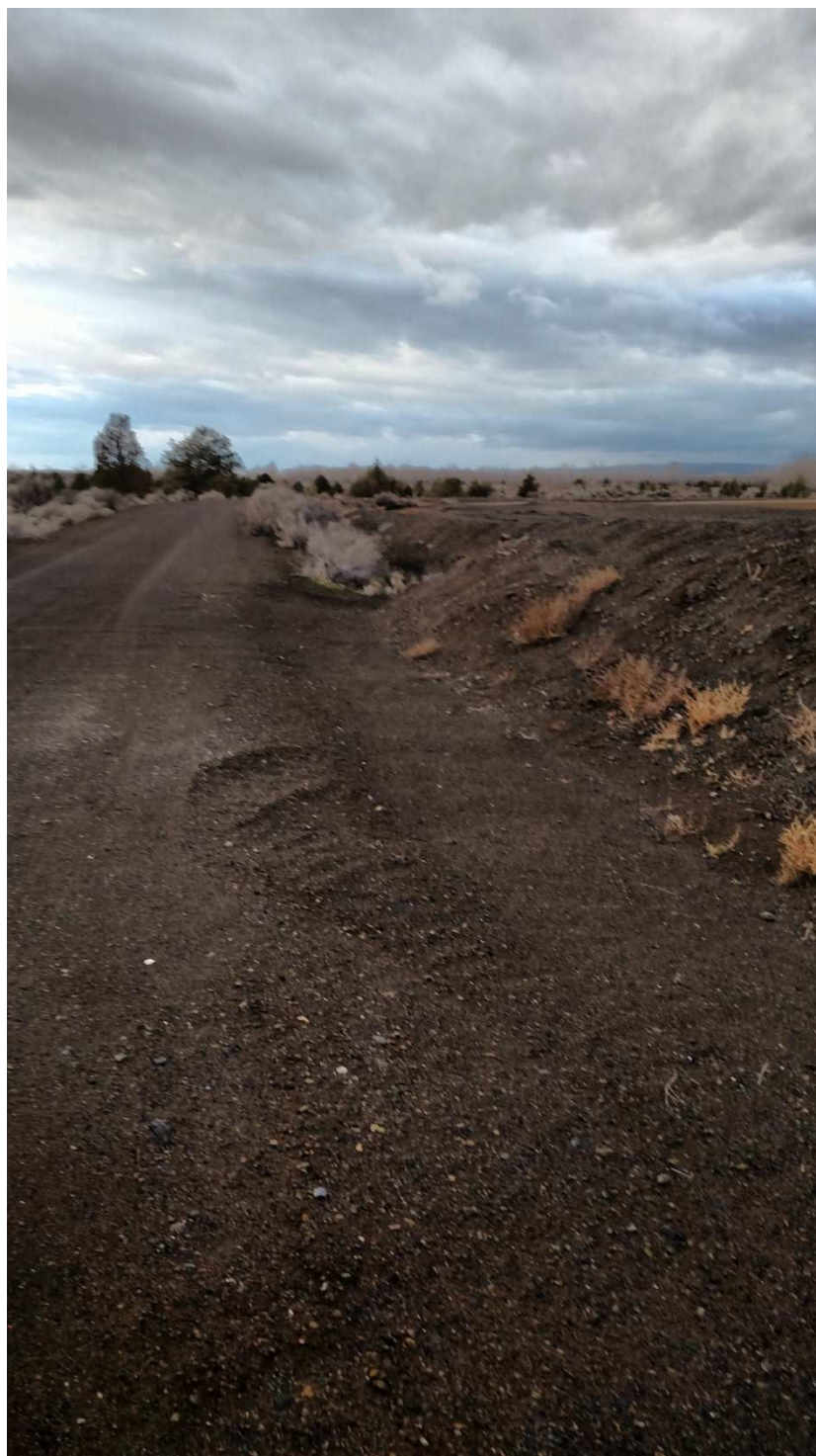
CCR landfill at south side, viewing west. South perimeter ditch.
