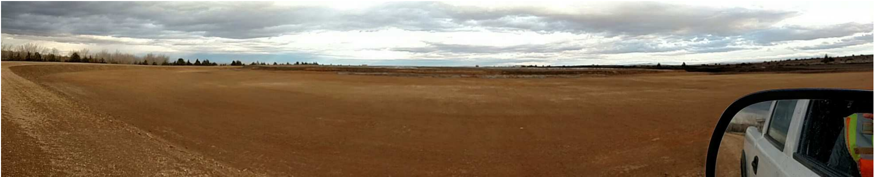
CCR landfill at west side, viewing east. Stormwater retention area.
