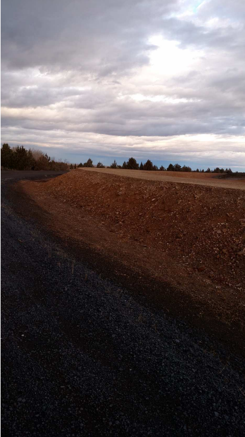
CCR landfill at west side, viewing northeast. Stormwater retention area impoundment.
