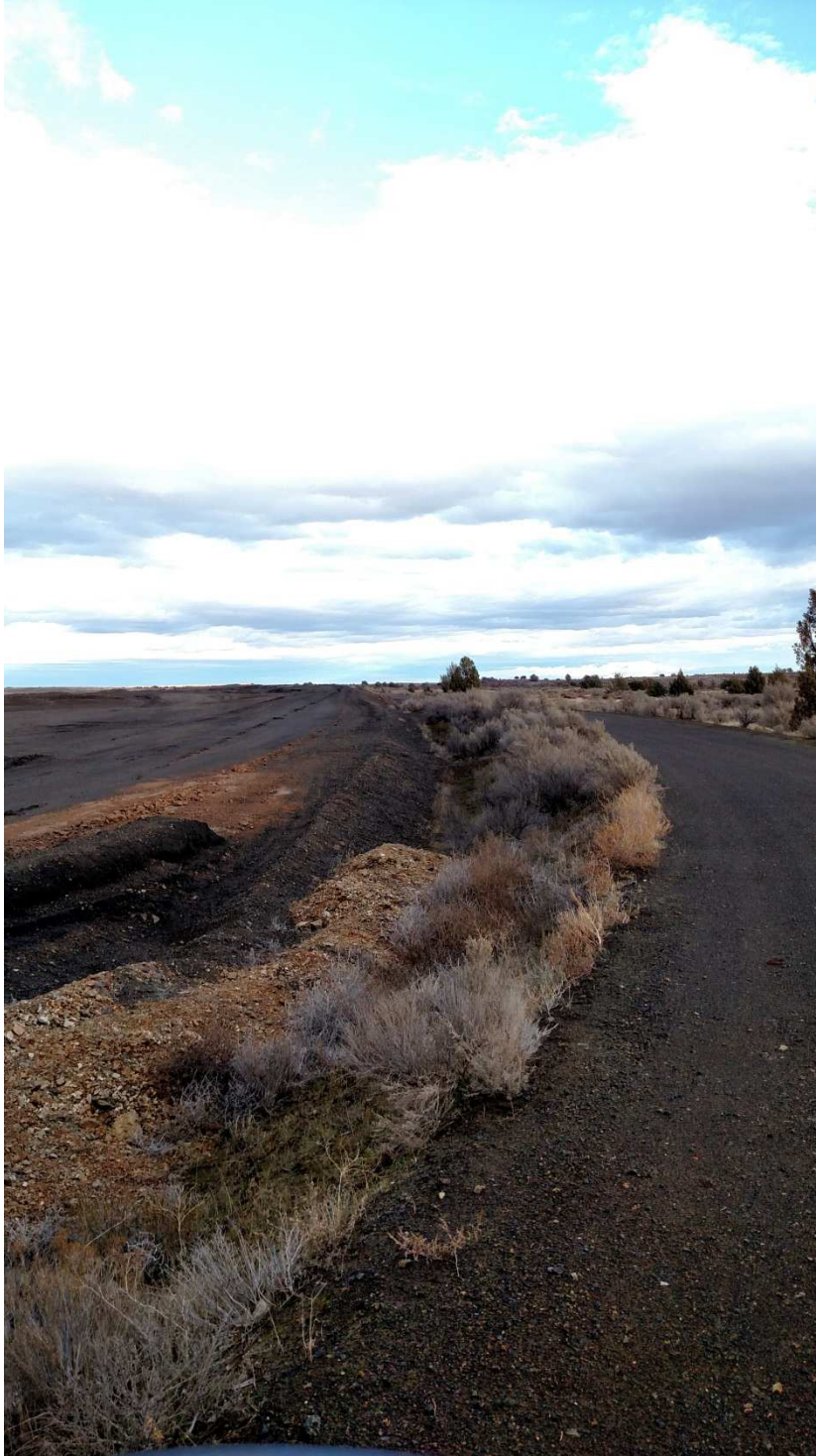
CCR landfill at southwest corner, viewing east. South perimeter ditch.
