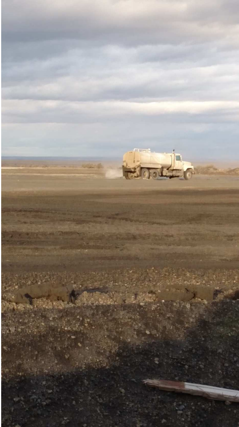
CCR landfill south side, viewing north. Water truck conditioning deposited fly or economizer ash.
