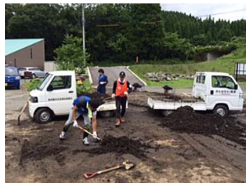
Employees digging up sediment
