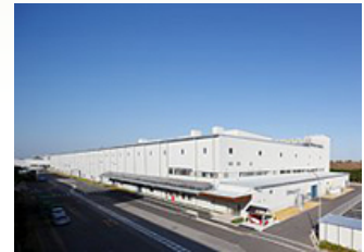
The waterborne paint Plant
