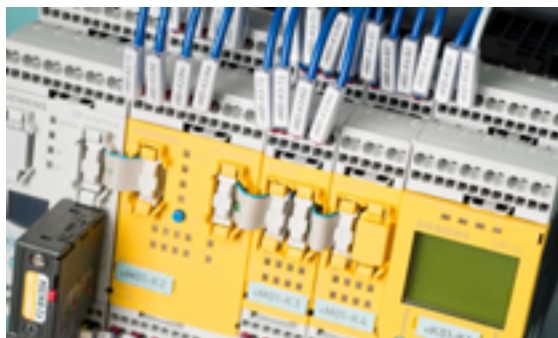
Figure 11-6 Example of conductor identification
