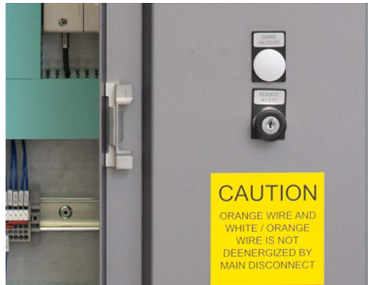
Figure 13-17 Example of safety sign for disconnecting means
