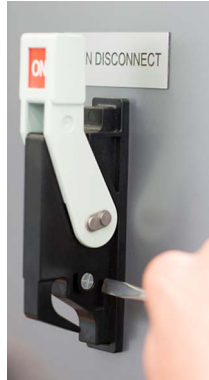
Figure 5-16 Example: Defeating with a screwdriver
