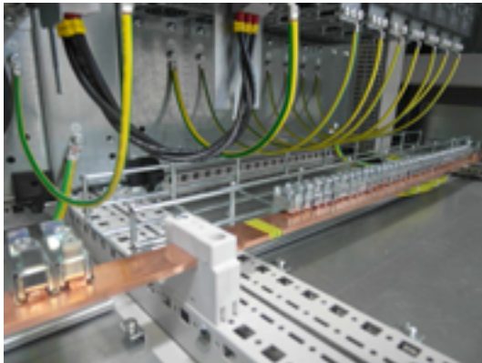
Figure 8-1 Grounding concept of an industrial control panel
