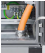
Figure 11-9 Cable entry example
