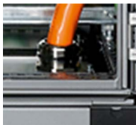
Figure 11-13 Cable entry through a connection receptacle (socket) in accordance with UL 514B
