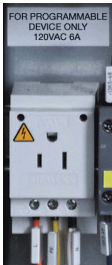
Figure 6-18 Marking of a receptacle
