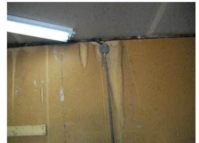
Water stains at the garage walls
